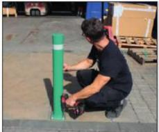
**4.** Fix the screws using a pipe wrench or screwdriver.
